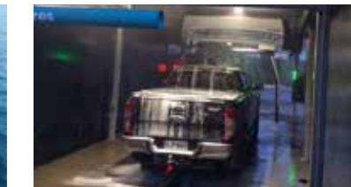
Connection of LED luminaires in a car washing plant (New Zealand). Series TH387.
